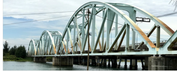
(b) Real view of the Nam O bridge
