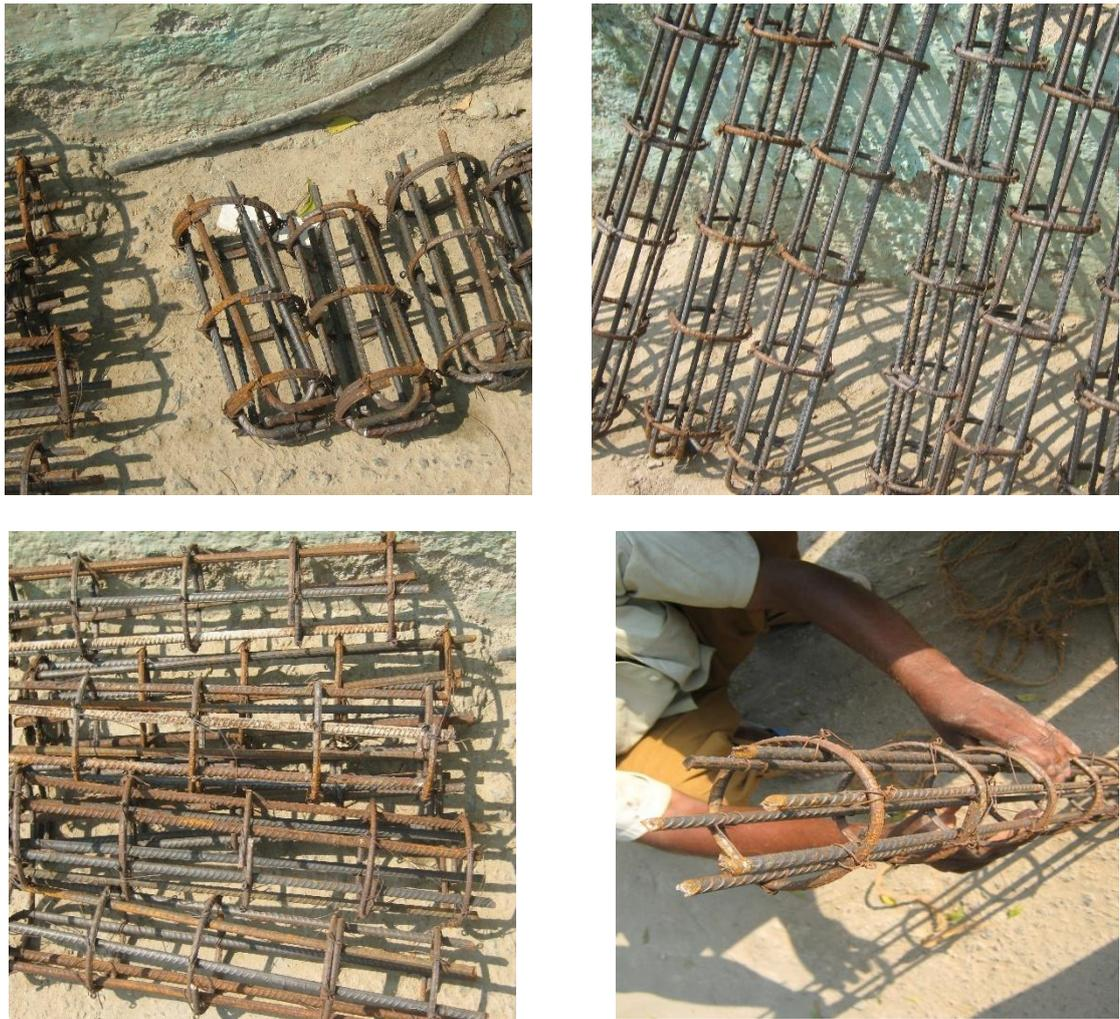
Figure 2. Steel reinforcement cage for casting the column specimens.
