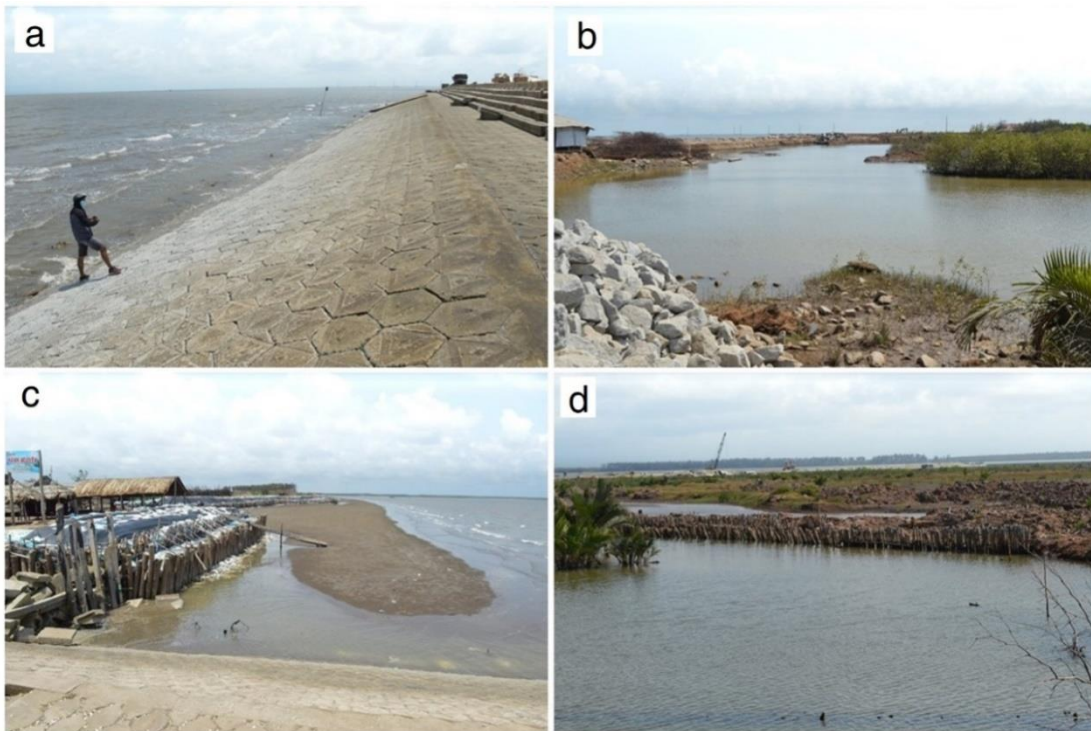
Figure 3. Hard structures (a-b) and breakwaters (c-d) used for coastal protection in Ben Tre.
