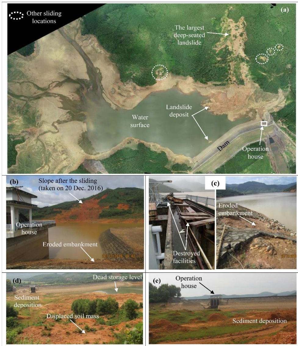
Figure 2. (a) UAV's photo of the Van Hoi reservoir, (b, c) Photo of the slope after sliding and its extensive damage to the dam facilities on December 20, 2016 (Photos courtesy by Do Canh Hao), and (d, e) Sediment deposition reservoir floor took on October 4, 2019
