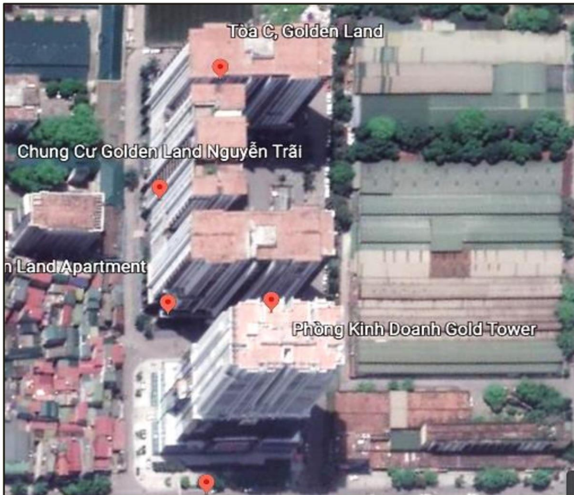
Figure 6. Golden Land building on Google Earth (a) and investigation in the field (b)
