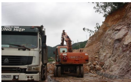
Figure 2. Handling landslides on Highway 18A in Cua Ong ward, Cam Pha city, July 8, 2017. (Source of photos: www.baoquangninh.com.vn )
