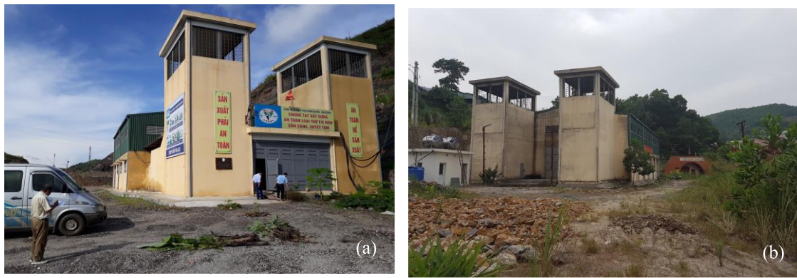
Figure 1. Main fan station - Design I: (a) 2K56-No.24 at East Wing and (b) 2K56-No.24 at Vu Mon, Mong Duong coal mine
