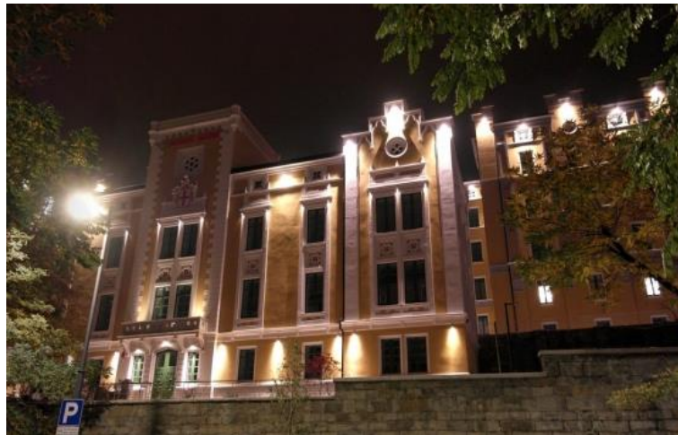
Figure 10. University College Luciano Fonda - Trieste. Seismic verification made before the inauguration of the student college can be summarized as follows: NDSHA (0.16g) compatible with standard (475 yr) PSHA (0.12g) at bedrock
