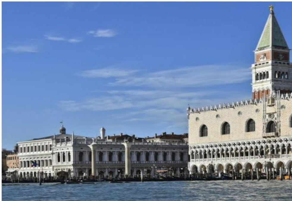
Figure 12. Marciana Library - Venice. The NDSHA study, performed in agreement with NTC 2008 and NTC 2018 chapter 3.2.3., has been supported by Segretariato Regionale of MIBACT. https://www.veneto.beniculturali.it/prevenzione-sismica-area-veneta
