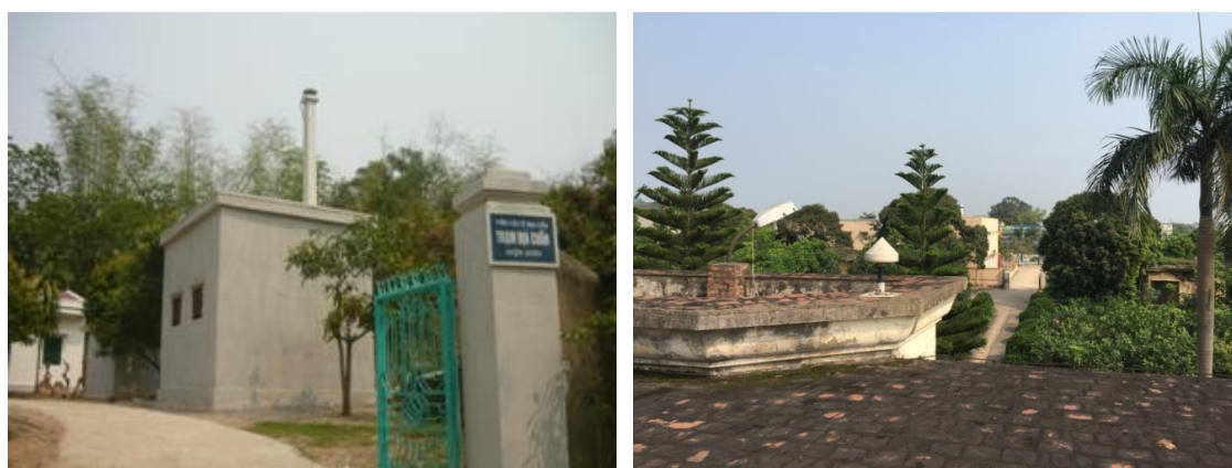
Figure 1. Antenna at the DBIV station (left) and at the PHUT station (right)
