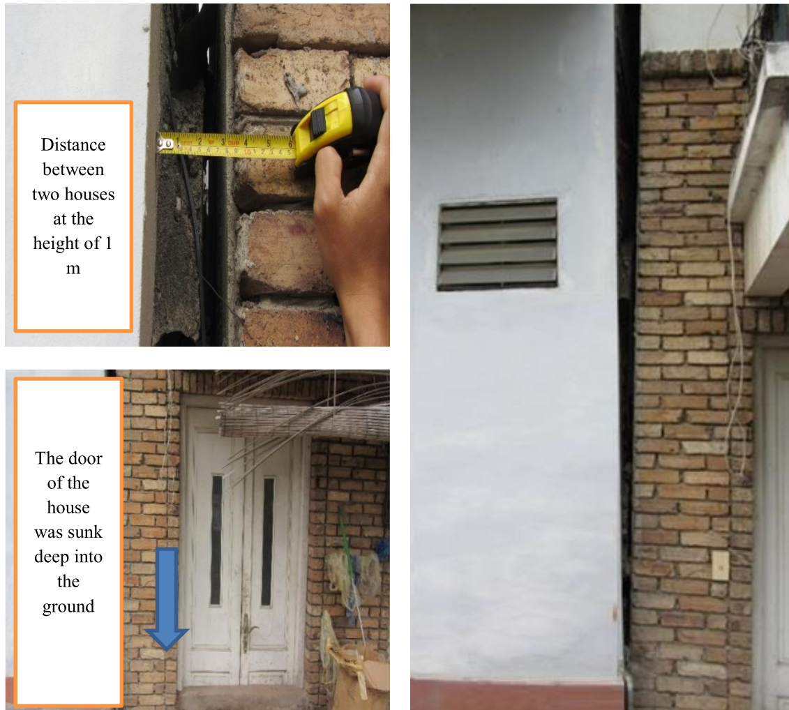
Figure 14. Serious subsidence threatens people's lives in Vinh Hung Ward, Thanh Tri ward, Hoang Mai District
