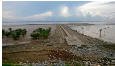
Trees grew in 2014 at left and right sides of groins A and B (growing in mass near to the foot of dyke)
