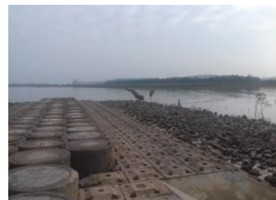
Bamboo stakes drove in sites of two groins in 2018
