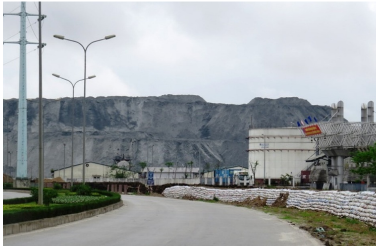
Figure 2. A “mountain” of untreated Gyps waste, polluting the environment from DAP-VINACHEM Joint Stock Company (Dinh Vu Industrial Park) - photo took in 2017
