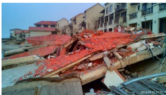
a) Large waves completely destroyed coastal buildings of Fusion Alya hotel [Photo taken on 16 April 2016]
