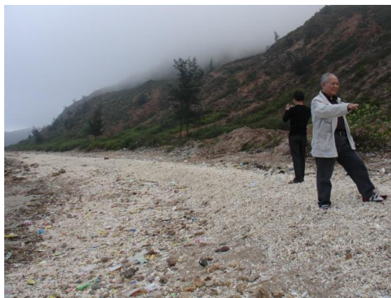
Fig. 4. Dyke, which consists of arca, snails mixed with pebbles along Lach Quen coastline of Quynh Luu district [Source: Cao Dinh Trieu (2011)]
